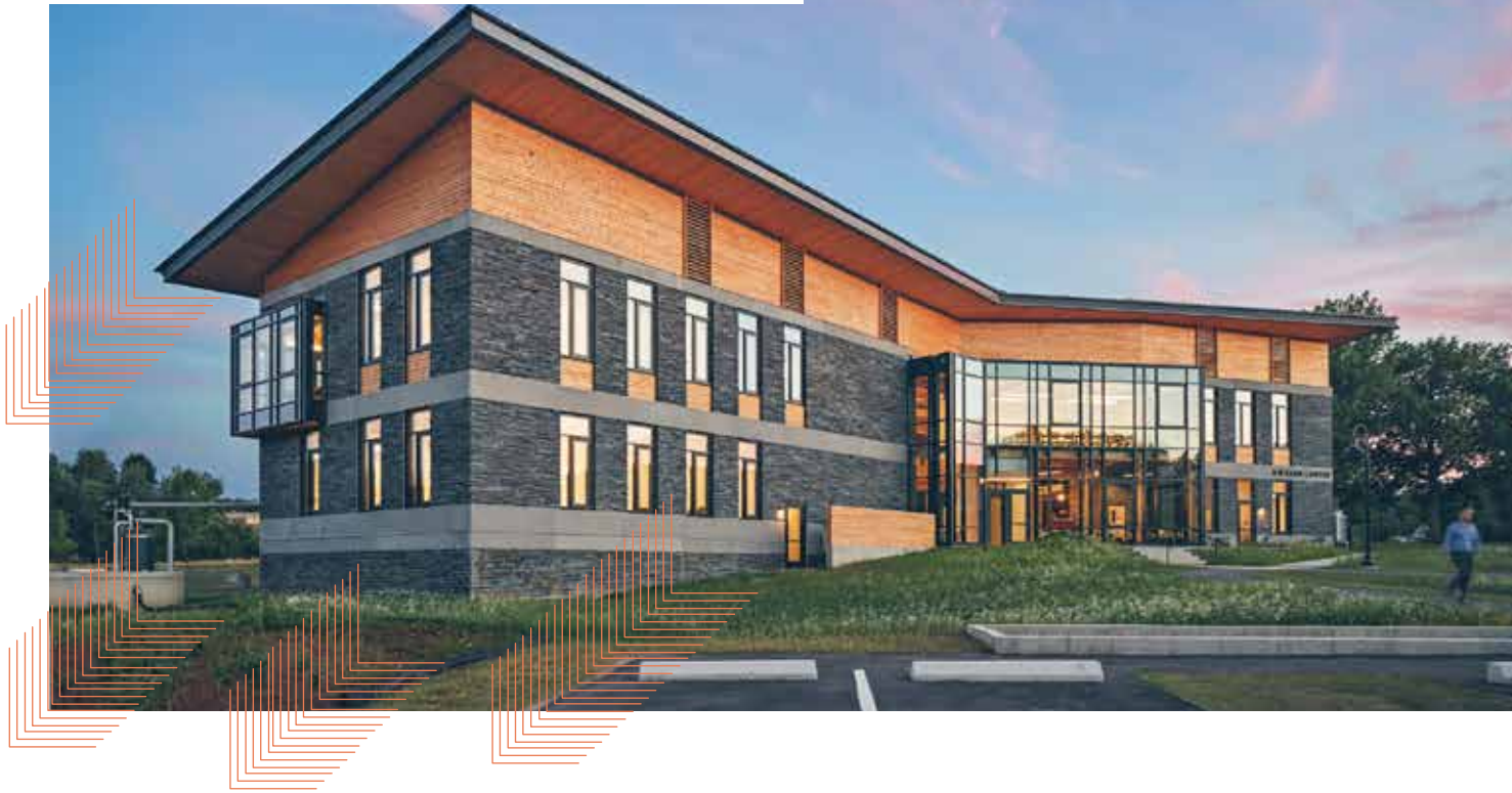
R.W. Kern Center, Hampshire College, Amherst, MA Building envelope protected, concrete flooring finished and exterior masonry protected with PROSOCO products
