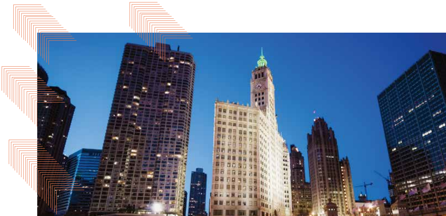
Wrigley Building, Chicago, IL Exterior terra cotta cleaned with PROSOCO cleaners and facade secured with PROSOCO anchors
