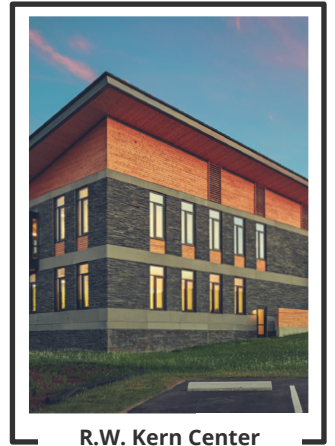
R.W. Kern Center at Hampshire College
